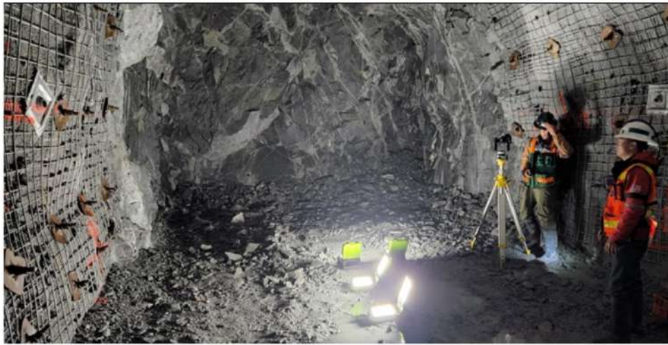
Figure 9. Photogrammetry data collection in underground tunnel
